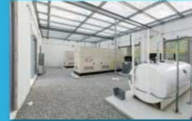
Fuel Storage / Generators
