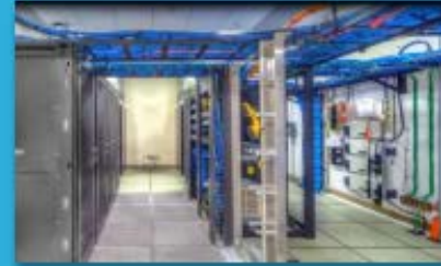
IT Server Room
