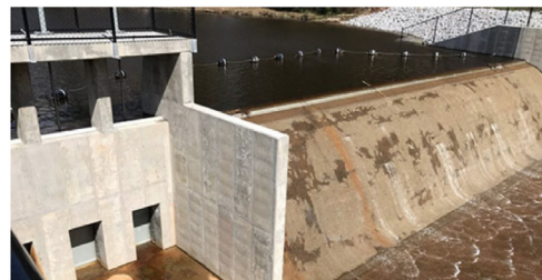
The rebuilt Cary Lake dam. Photo courtesy of Peter Chesney.
