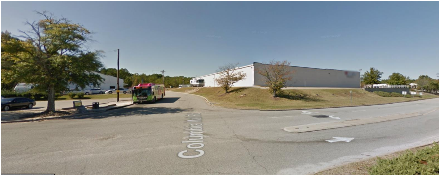
Image 2. Northeast Protection Connection Zone
