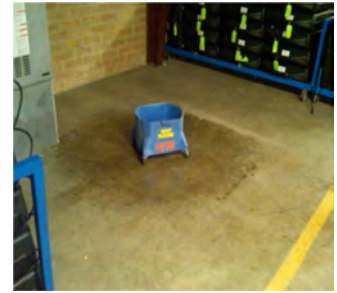
Elections & Voter Registration Warehouse Water Leak
