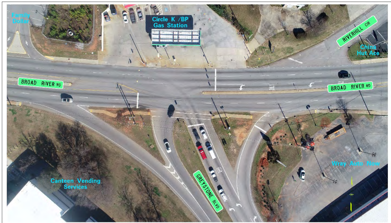
AERIAL VIEW OF INTERSECTION OF GREYSTONE BOULEVARD AND BROAD RIVER ROAD
