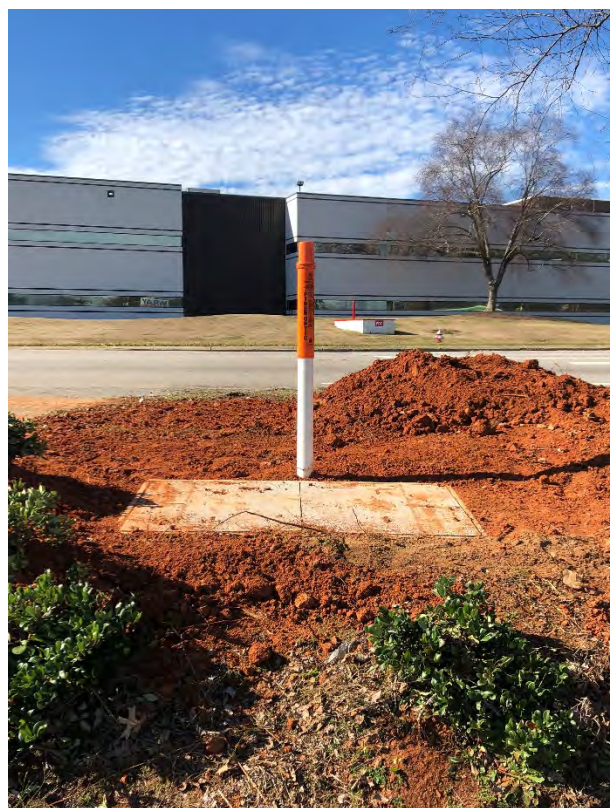
RECENT INSTALLATION OF FIBER OPTIC VAULT AT GREYSTONE
