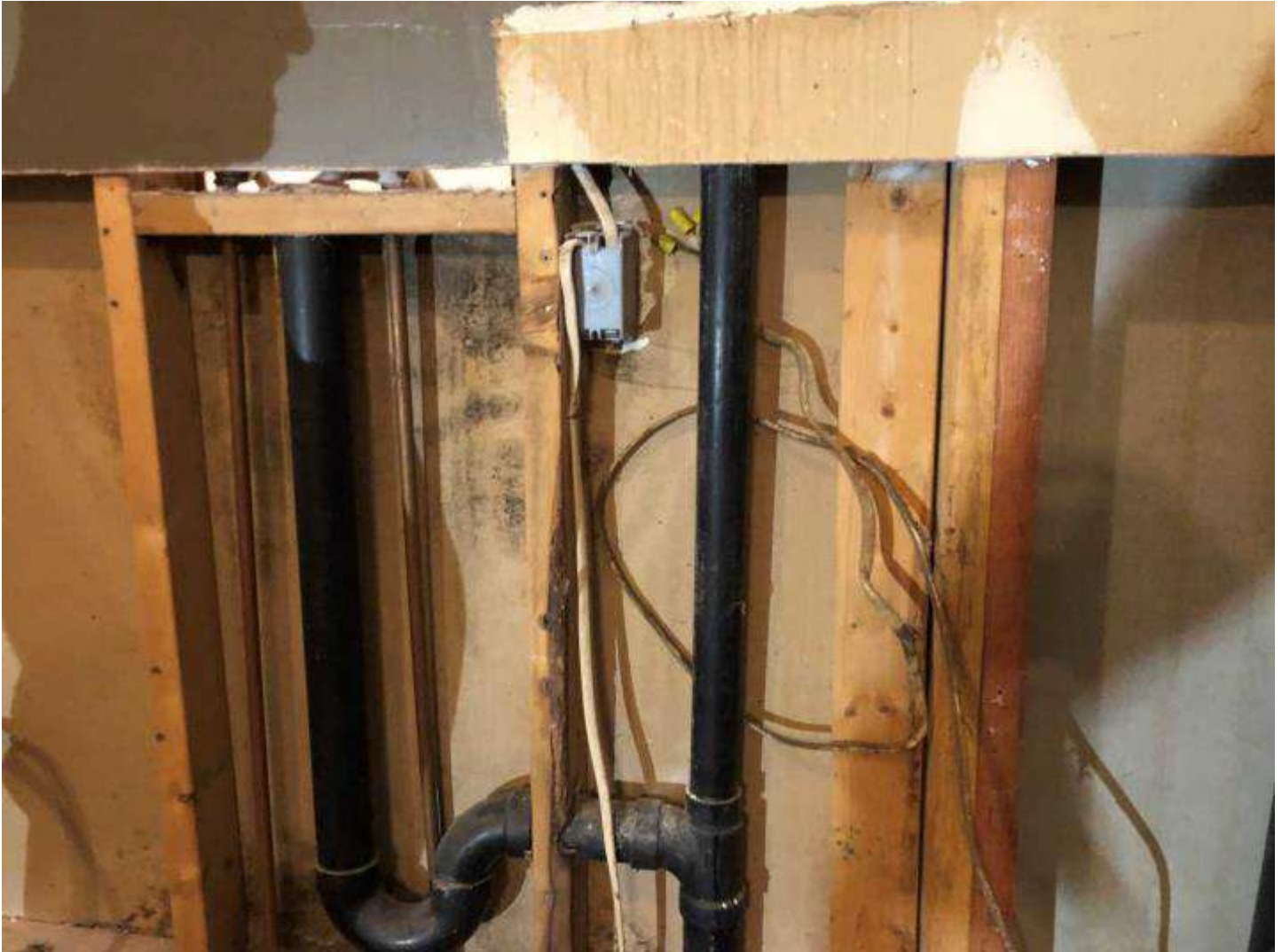
4 4-IMG_3309 Date Taken: 5/27/2020 one of the wires that were laying in the crawlspace . it did not even have wire nuts on it either.
