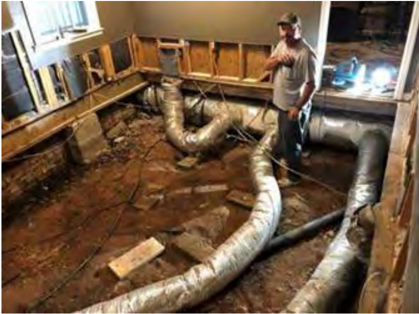
Picture 3: Shows the contractor able to observe past the duct work into the den upon removal of the floor joists in the kitchen and identify the issue with the floor joists in the den.
