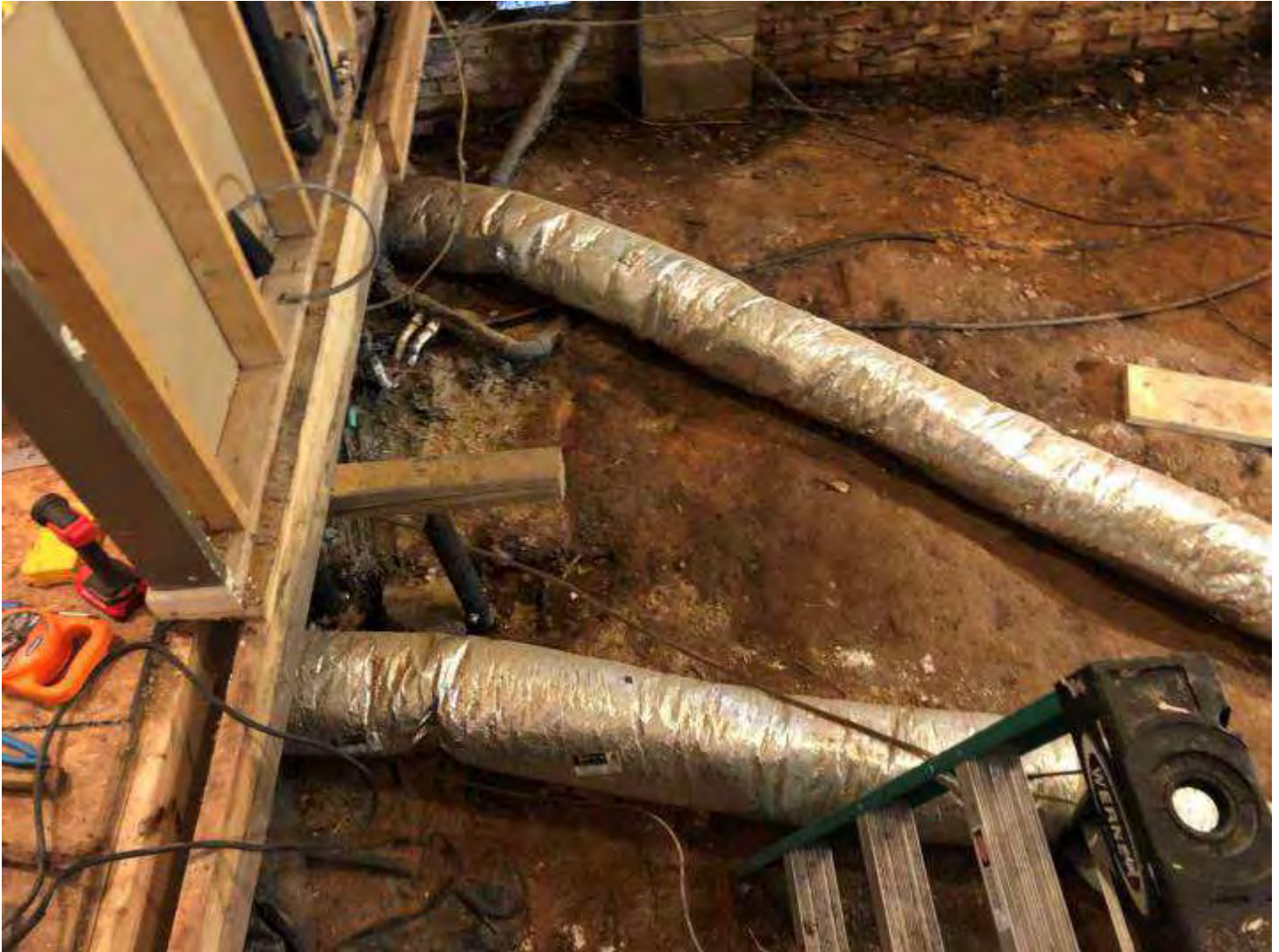
3 3-IMG_3308 Date Taken: 5/27/2020 old repair work were someone attempted to use floor jacks that just sunk into the ground.
