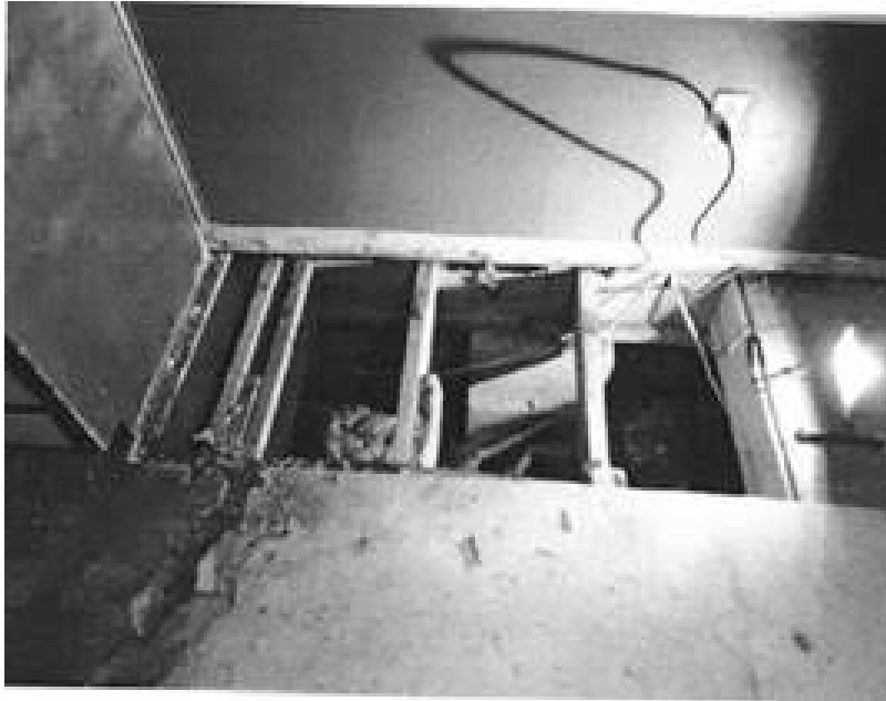
Picture 1: Shows the joist issues identified for Change Order #1.
