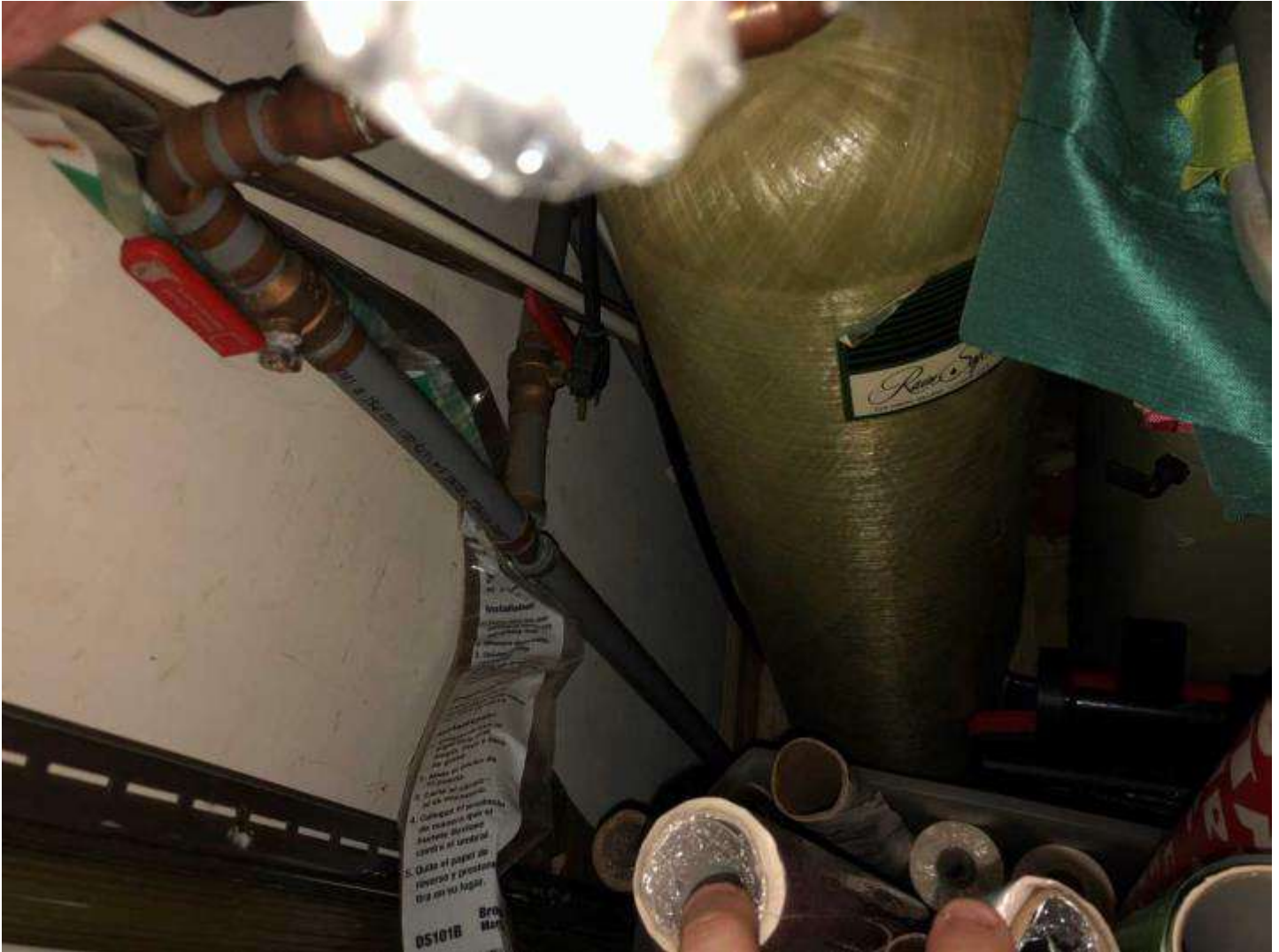
10 10-IMG_3315 close up.
