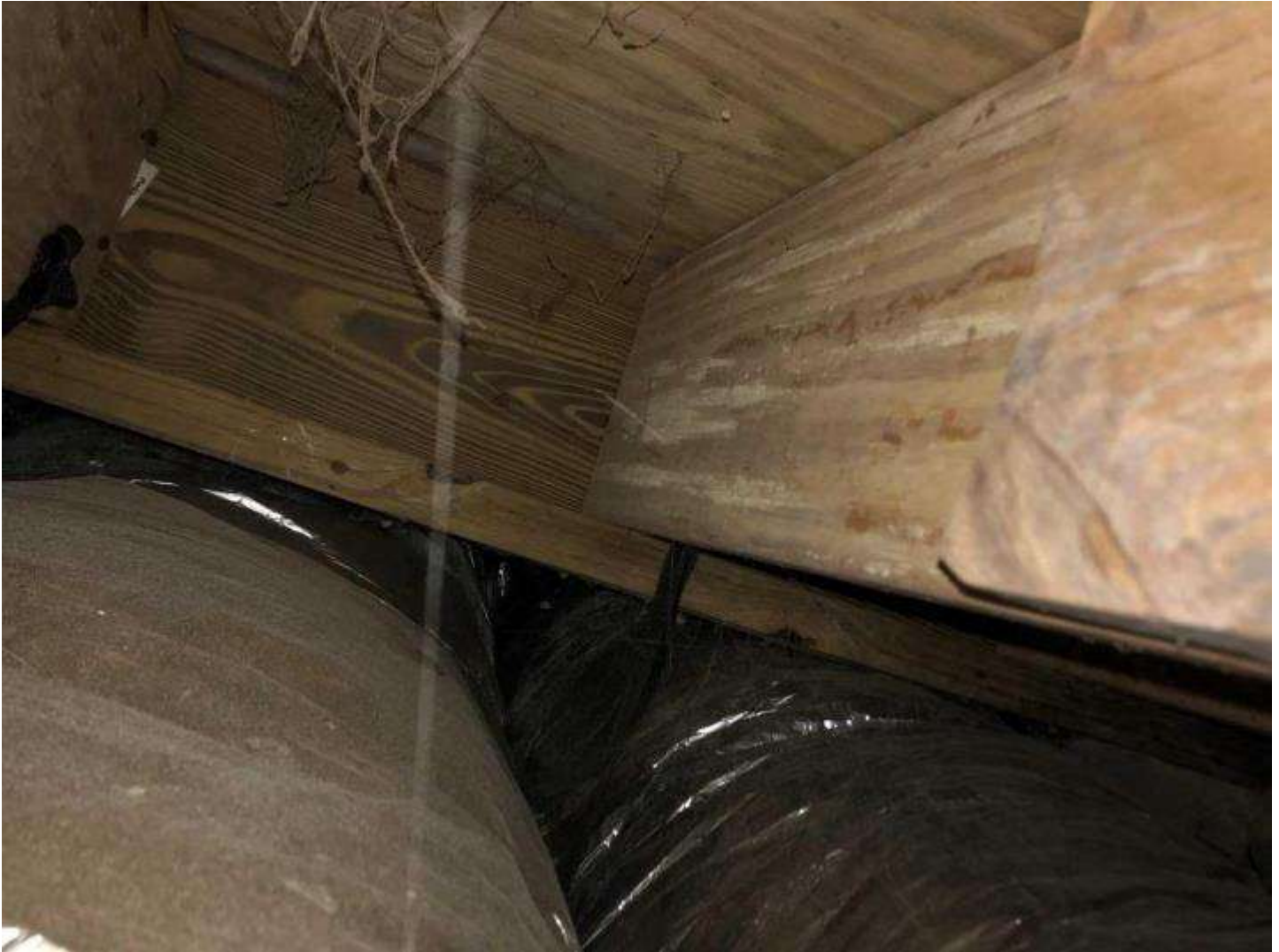
15 16-IMG_3321 Date Taken: 5/27/2020 also they are NOT nailed into the seal.
