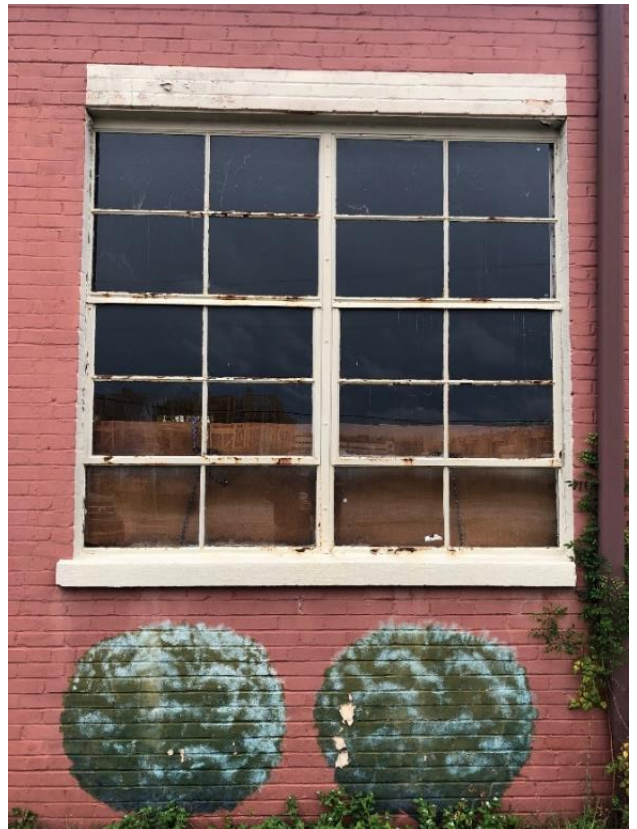
Steel casement window
