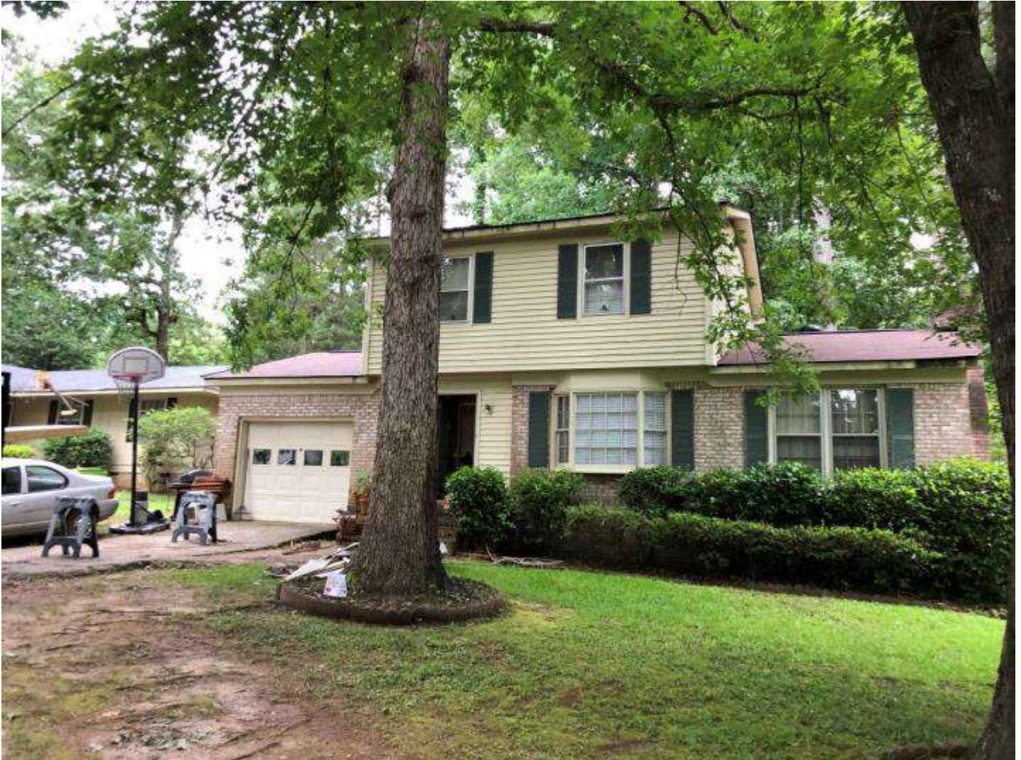
1 1-IMG_3306 front of the residence
