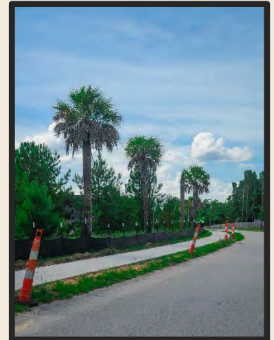
Harrington Road Sidewalk construction is underway.
