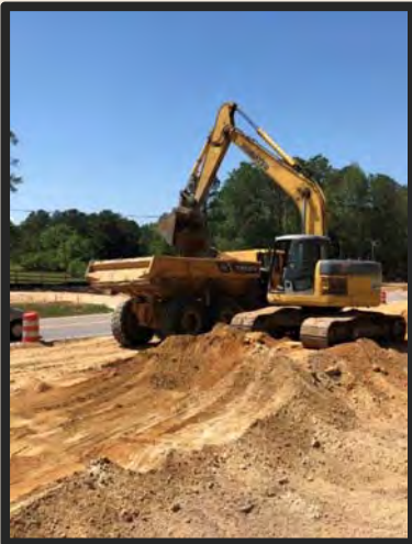
Progress on the Hardscrabble Road Widening project.
