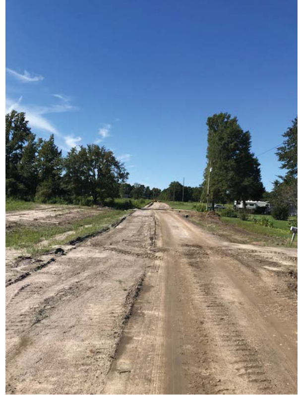
SOUTH DRIVE DIRT ROAD PAVING
