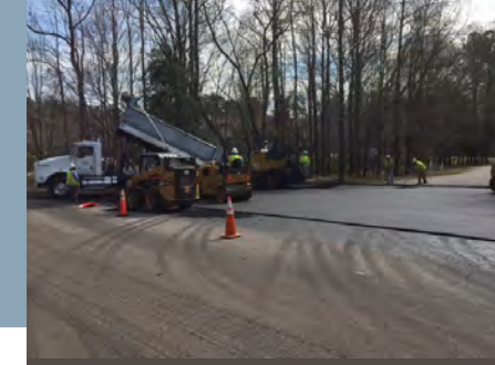
Resurfacing Finley Road
