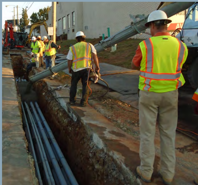
North Main Street Widening
