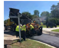
Cove View Drive Resurfacing Project
