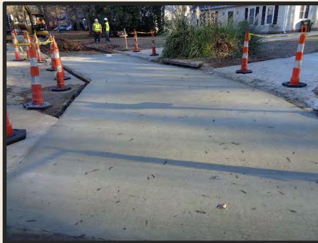
*Concrete patching on Lyne Cove Court, one of 81 roads being improved under the Resurfacing Package "P" contract.*
