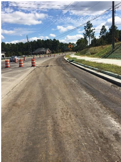
Clemson Rd. Roadway Widening
