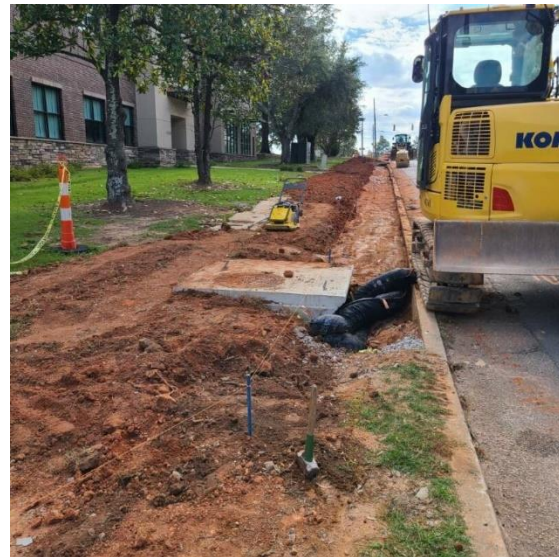
N. Main St. Sidewalk Installation
